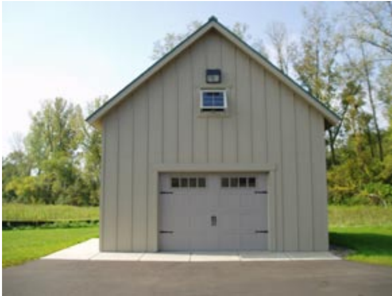
New Small Storage Building
